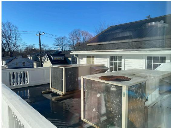
FPB's 1999 rear addition has four HVAC zones, defined by the ductwork in the walls and ceilings. Each zone is heated or cooled by a Roof Top Unit (RTU) powered by electricity (AC) or a combination of natural gas and electricity (heat). Until late 2024, all four RTUs were original. But at the end of 2024, the RTU with the most load (i.e. hours) had a corrosion failure that could not be repaired cost-effectively.
